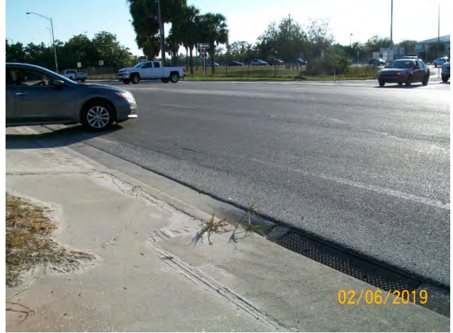
Photo 2-6: Vehicles exiting Structural Steel entrance onto northbound 31 st Street are conflicting with vehicles attempting to U-turn from right lane of off-ramp
